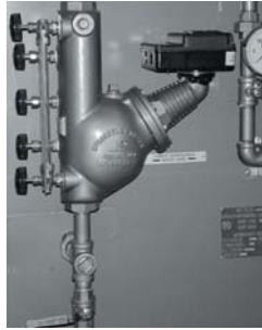
Float Type Pump Start/LWCO
