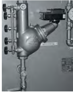
Float Type Pump Start/LWCO
