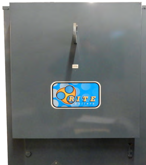
INSULATED HEAD PLATE COVER INSTALLED
