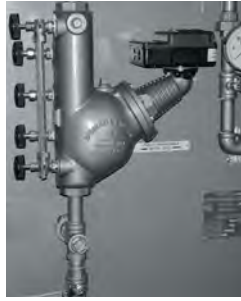
Float Type Pump Start/LWCO
